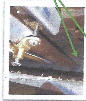
Pipe coming through floor
